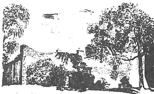
Buchanan Castle Golf Club House contains part of the ancient remains of the Place of Buchanan.
